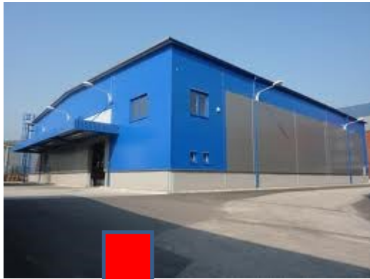
Storage hall (Location)
