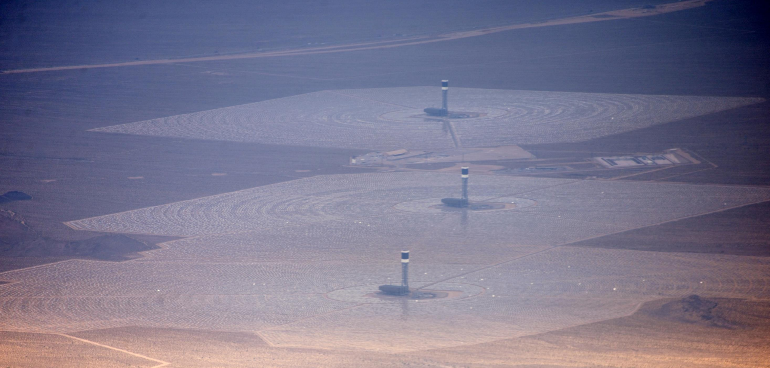
Ivanpah I, II, III Solar Electric Generating System, Ivanpah, California, USA (123 + 133 + 133 MWe)
