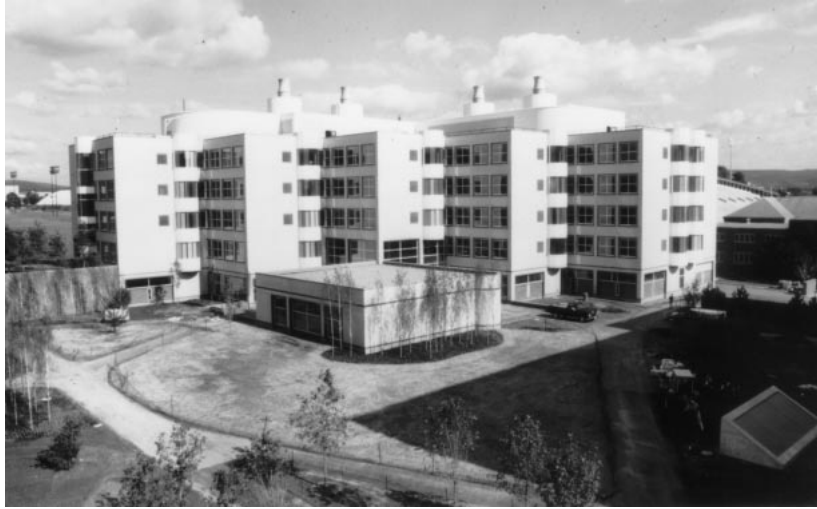
Figure 1. Exterior view of CBB.
