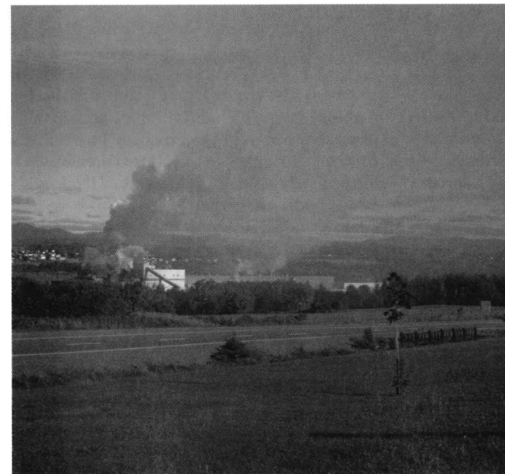
Figure 21-7 Industrial pollution. Because the stack of this wood-products mill in New Richmond, Quebec Province, Canada, lacks electrostatic precipitators, the plume contains substantial amounts of suspended particulate matter that can be seen from a great distance.
