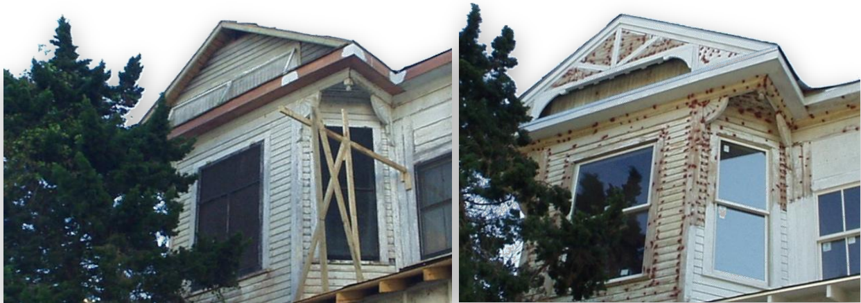
Figure 19. Windows and Trim , April 8, 2003 and January 3, 2006 (photos by the author).
