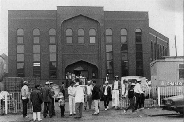
Fig. 1. The Al-Bukhari Mosque, Loughborough Road, Opened in 1985 and was the Second Purpose-Built Mosque in Leicester ( Leicester Mercury ).
