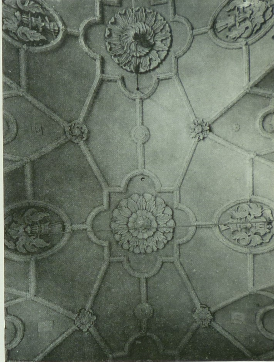
334 Jan Jaroszewicz and Jan Wolff: Vault decoration, painted stucco, about 1625. Uchanie, Parish Church
