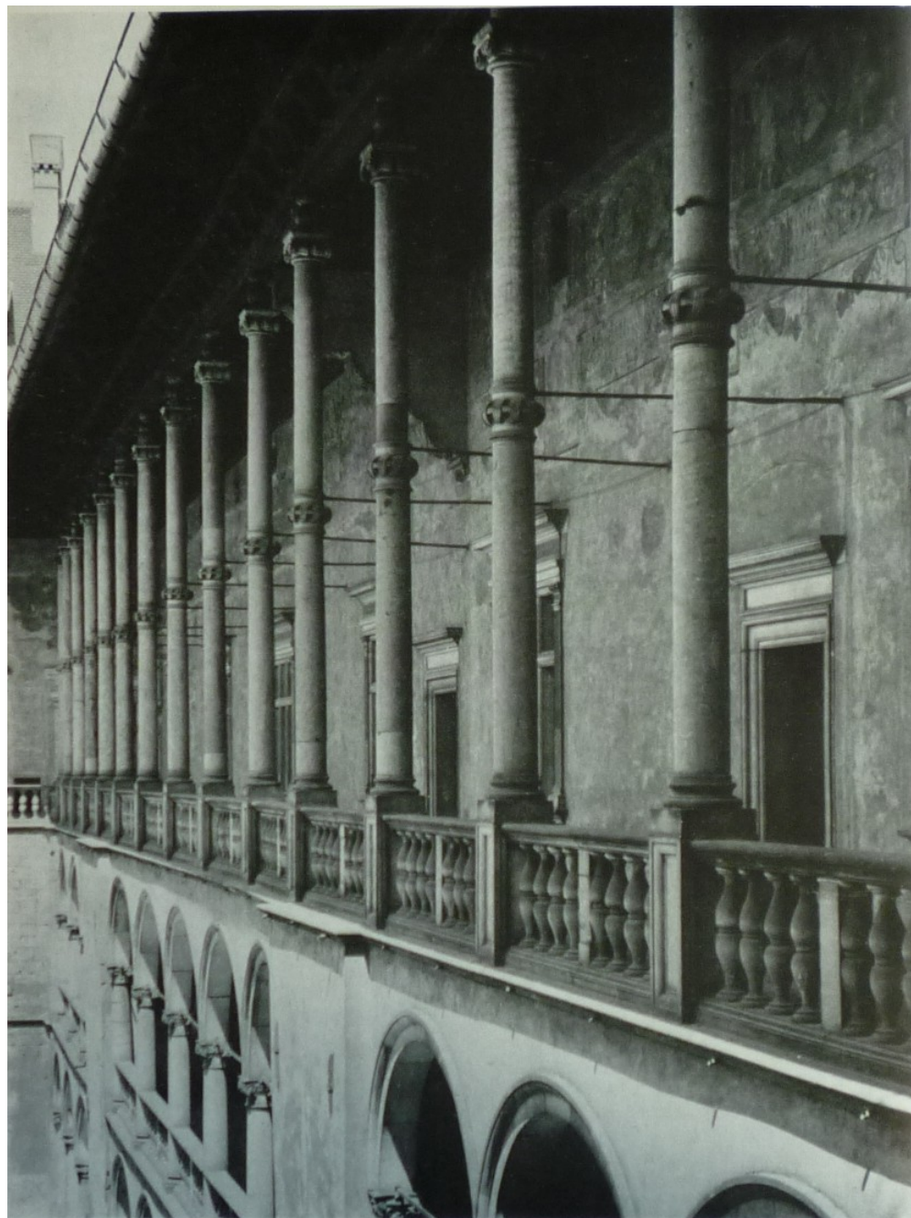
64 Columns of the upper floor arcade, capitals and coffered ceiling. Cracow, Wawel Castle
