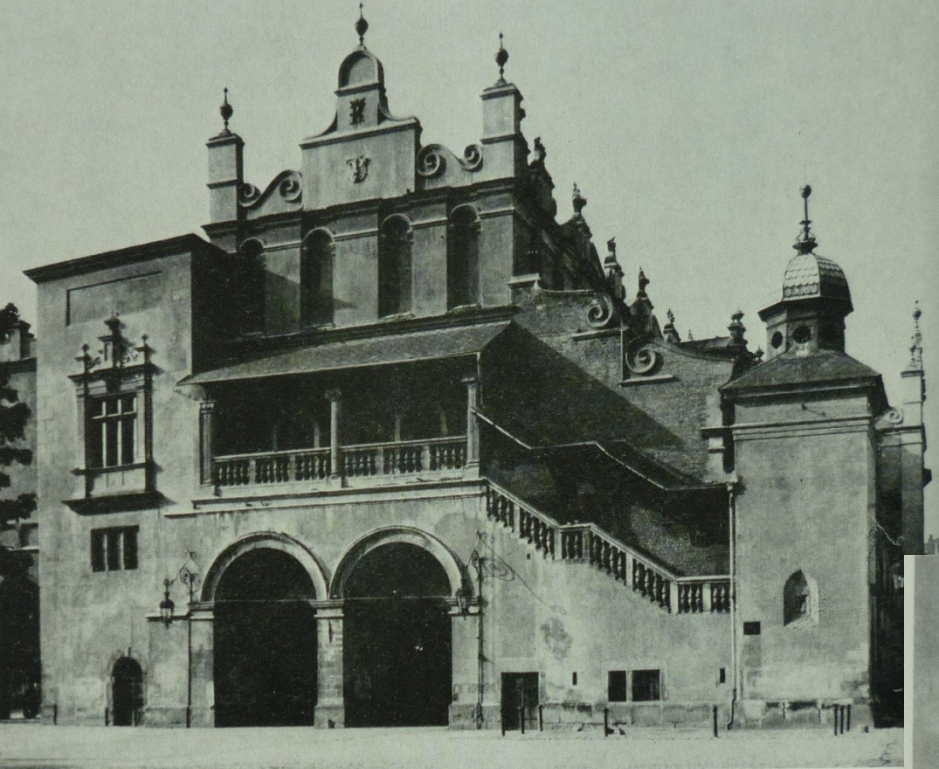
241 Cloth Hall. Short side from the south, probably by Gian Maria Mosca il Padovano. Some alterations of 1875-9. Cracow
