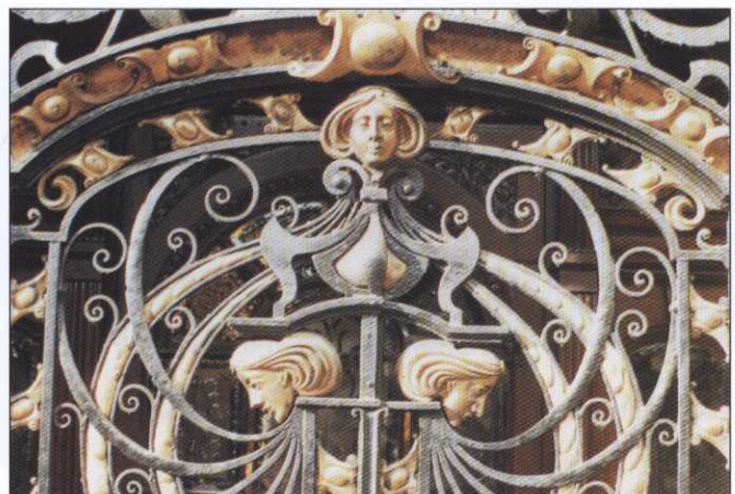
Gate, The Liverpool Philharmonic Hotel, Liverpool, England (1900) Iron and copper
