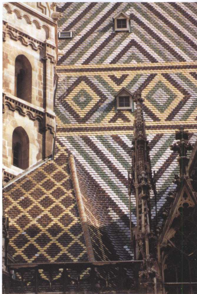
St. Stephen's Cathedral Roof, Vienna, Austria
