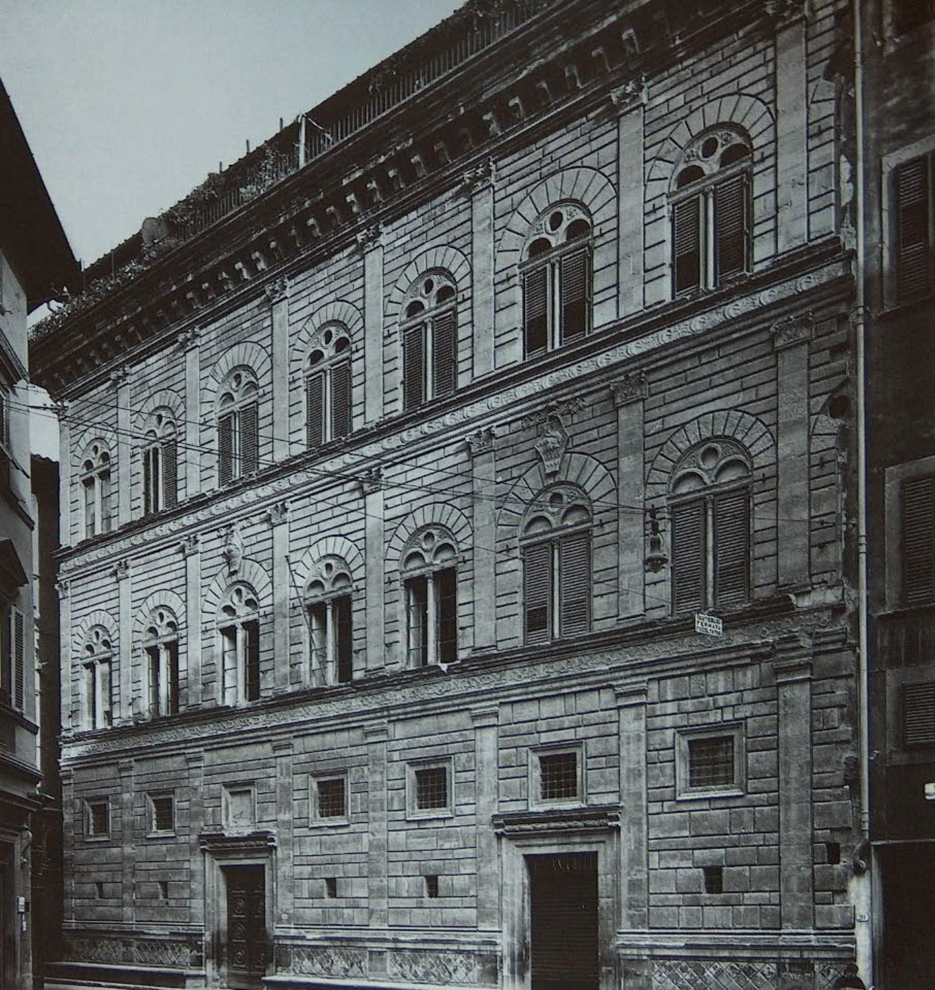
Florence, Palazzo Rucellai, po 1455-1470
