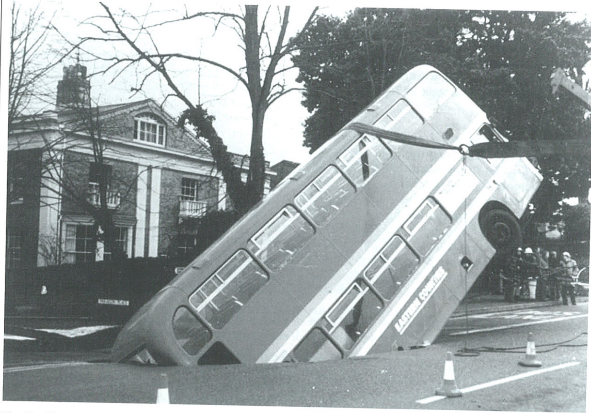
Fig. 10 Norwich. Subsidence due to flint mining, Earlam Road (Norwich City Council).
