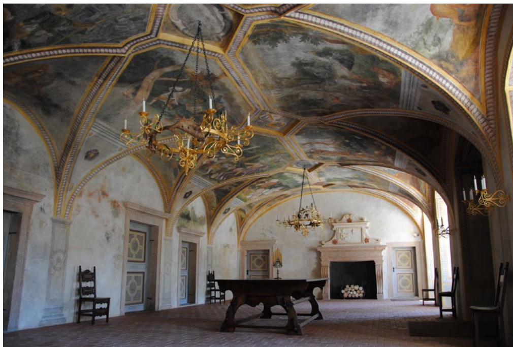
Fig. 6. Main floor entrance hall with fresco decoration depicting hunting scenes and themes from Ovid (Georg Widman from Brunswick, around 1590).
