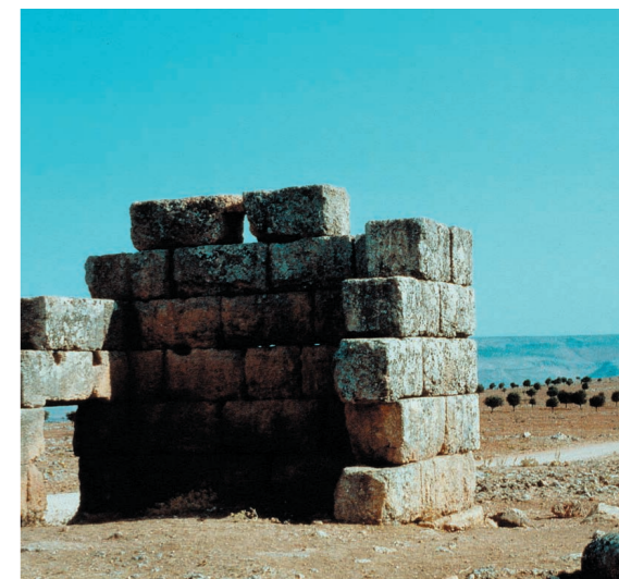
35. Towers, such as this one in Turkey, aided communication along the frontier roads
