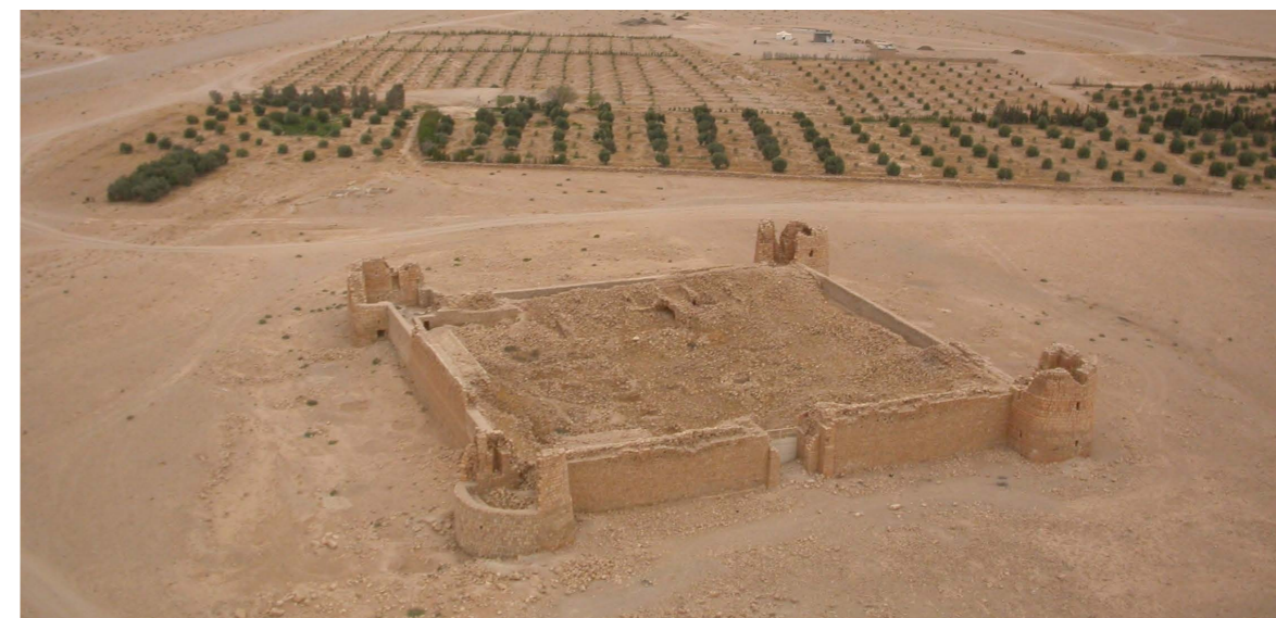
40. The military fortification at Hân al-Manqûra (Syria), probably dating to the middle of the second century AD 40. Vojno utvrđenje u Han al-Mankouri (Sirija), datuje se verovatno do sredine II veka n.e.
