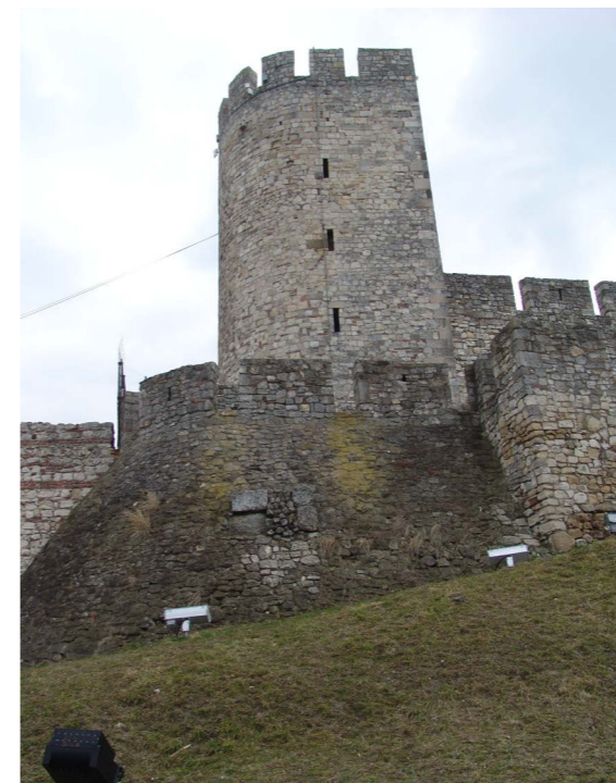
94. Singidunum - Remains of the late Roman wall of the Lower City incorporated into mediaeval fortification 94. Singidunum - Ostaci kasnoantičkog bedema Donjeg grada prekriveni srednjevekovnom eskarpom
