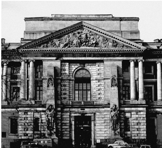
Fig. 5. Mikhailovskii Castle. Main Façade. Brumfield. 10/4/1984
