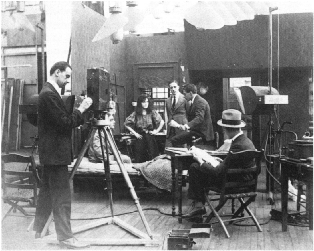
20.15 (opposite below) Cameraman Ned Van Buren filming in the Edison studio with a Moy camera, with director John Collins seated on the bed railing talking to the actors. Diffusers hang below the glass roof, while hanging enclosed arcs and broadside arcs on floor stands provide additional light
