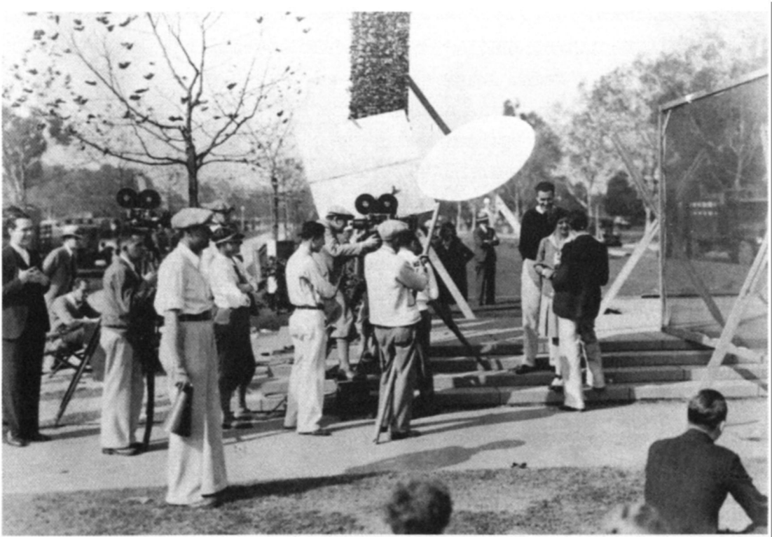
21.4 (below) Shooting a scene with Joan Crawford for Duke Steps Out (James Cruze, 1929, MGM). The Bell & Howell camera at center has a long lens and has been moved back to get a soft look, in combination with the diffusion disk overhead and diffusion screen behind the couple
