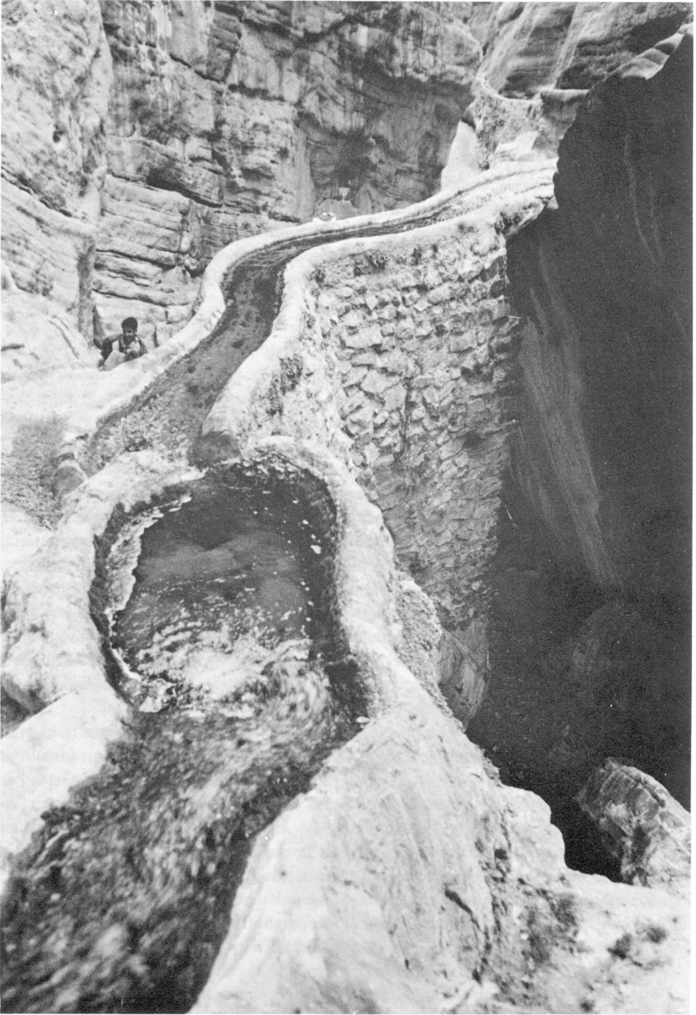
Plate 1 Falaj in the mountains of Wadi al Hijr. A flow-regulating tank.
