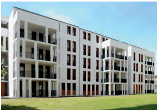
Leibar & Seigneurin Architects. Baiona
