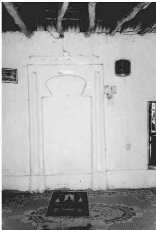
Figure 4.9. A simple Ibadi mihrāb in a small contemporary mosque at Tumbe (Pemba Island). The niche is marked in plaster, but no recess is in the wall
