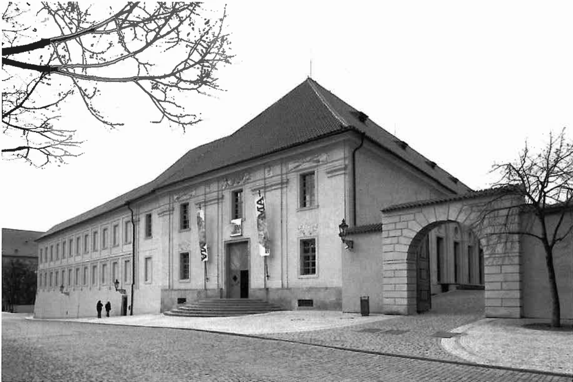
3. The Royal Riding School by Prague Castle, the front facing the street and the entrance to the Riding Hall (1694-1699). Photo: Martin Mádl.
