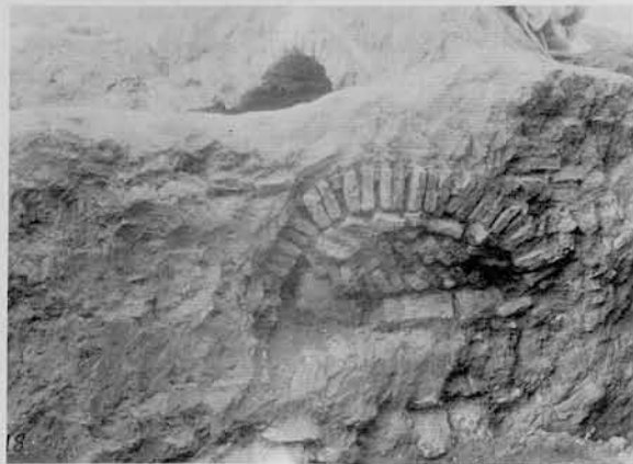
11 RT. 789: the southeast wall of the tomb-chamber from the outside showing the arched dome and door blocking of brick and stone and the collapsed vault behind.
