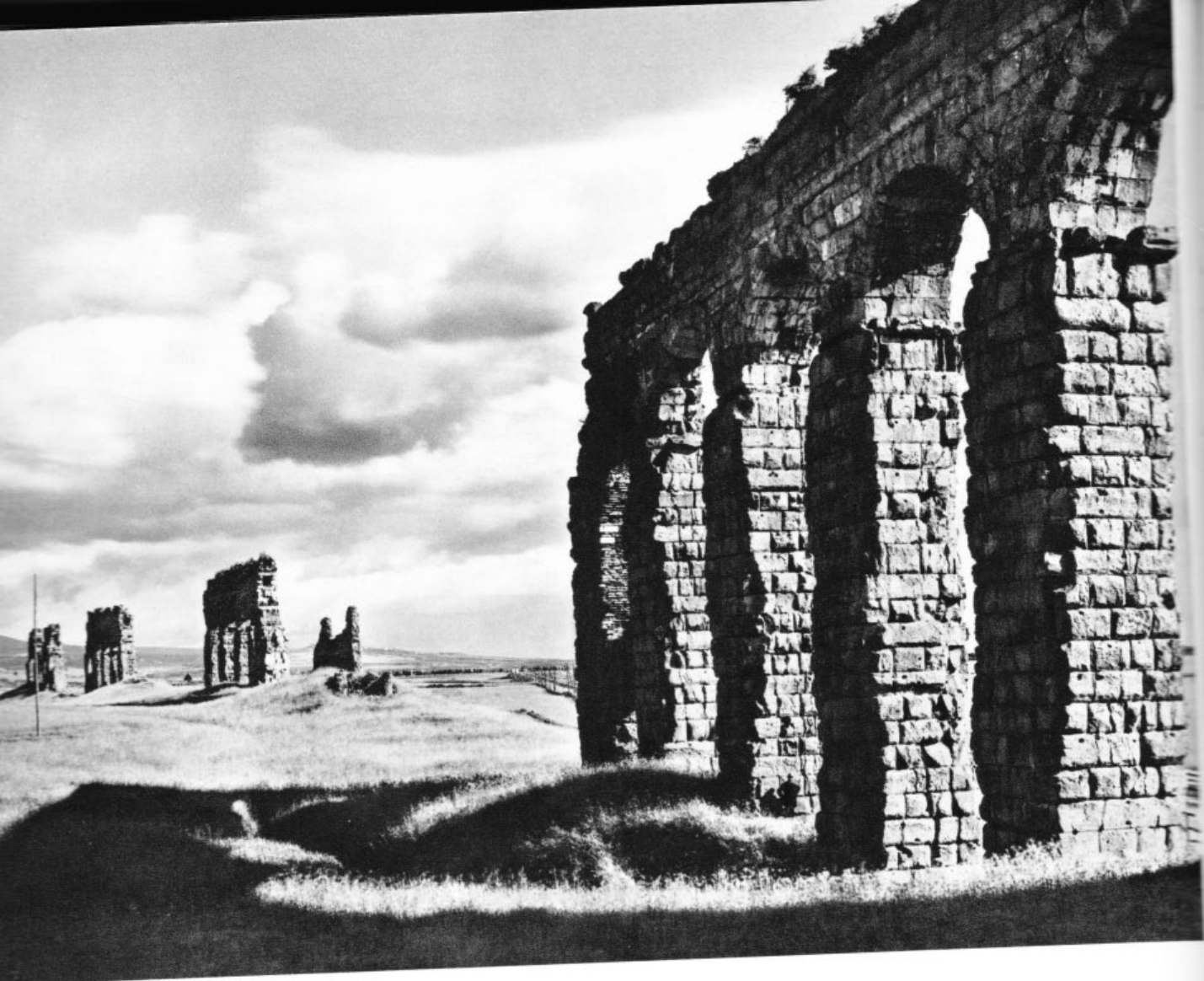
170 RUINS OF THE CLAUDIAN AQUEDUCT, NEAR ROME
