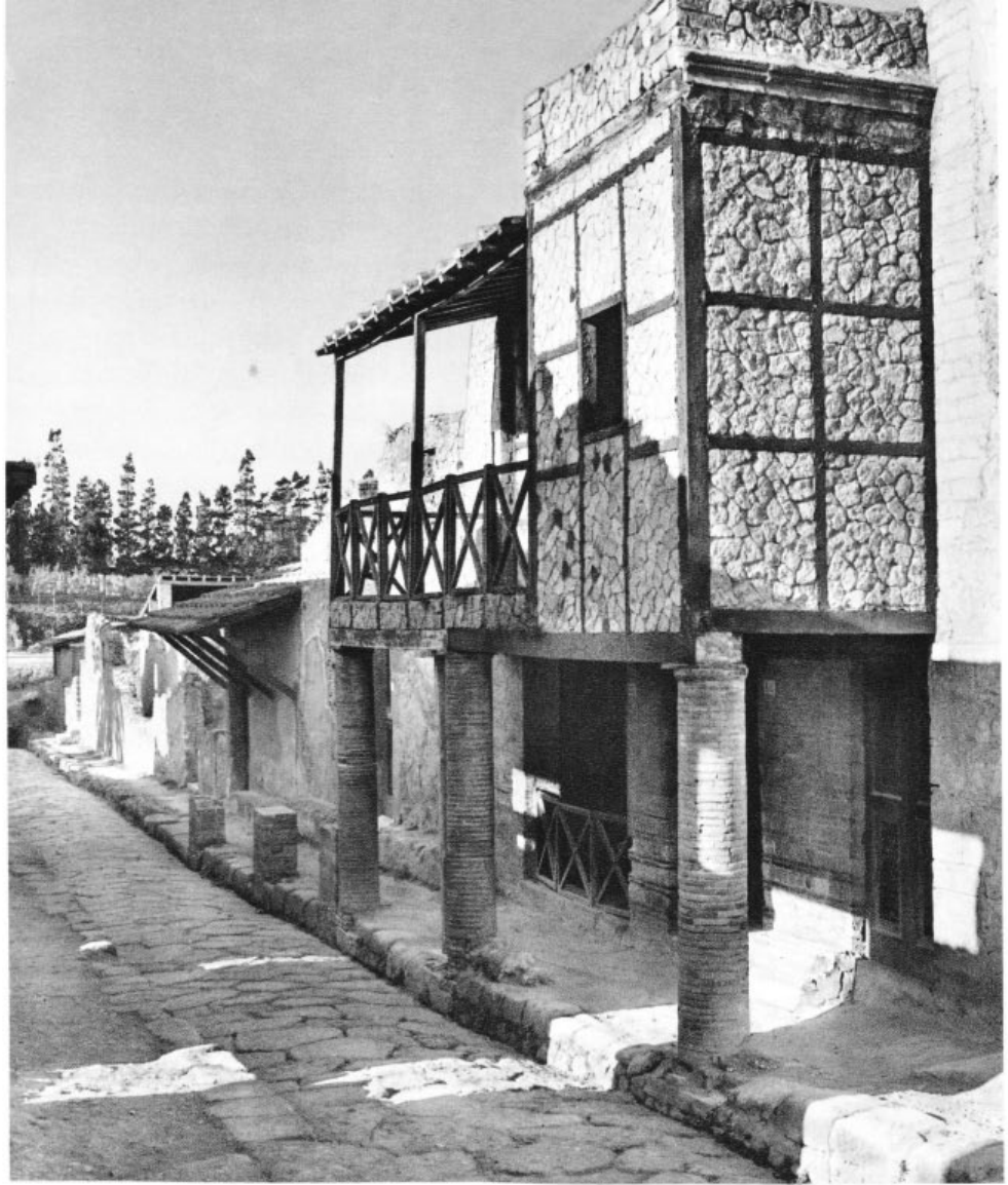
44 HERCULANEUM: HOUSE WITH WOODEN FRAMEWORK
