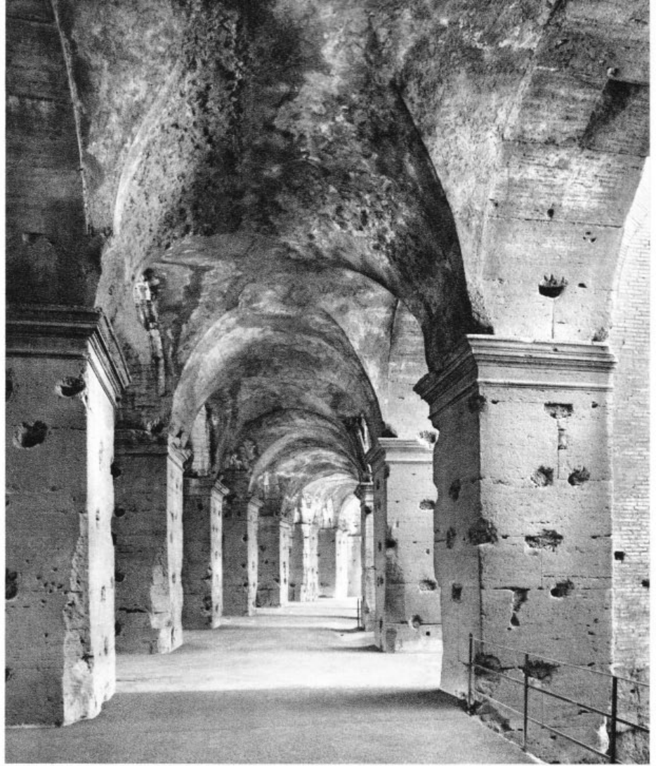
179 ROME, THE COLISEUM. FIRST-FLOOR CORRIDOR
