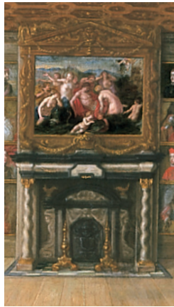
Fig. 13 Chimney in back room, after restoration
