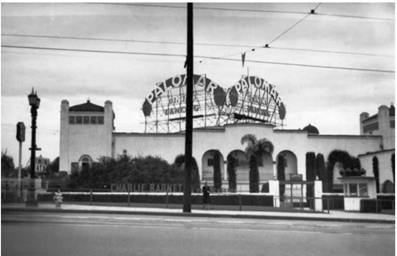
Palomar Ballroom, Vermont Avenue, Los Angeles
