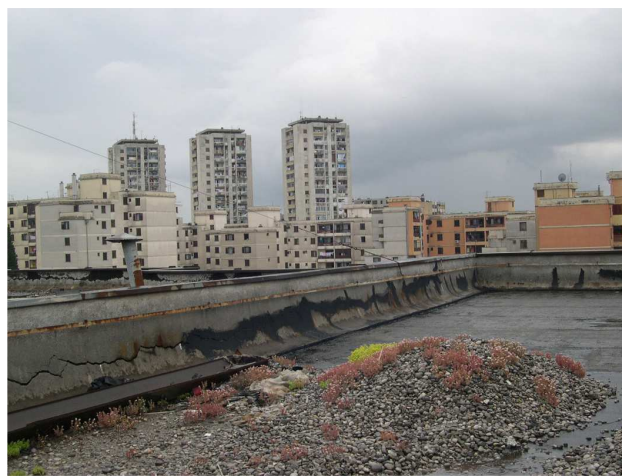
Figure 65. Building of Ei Niš (roof).
