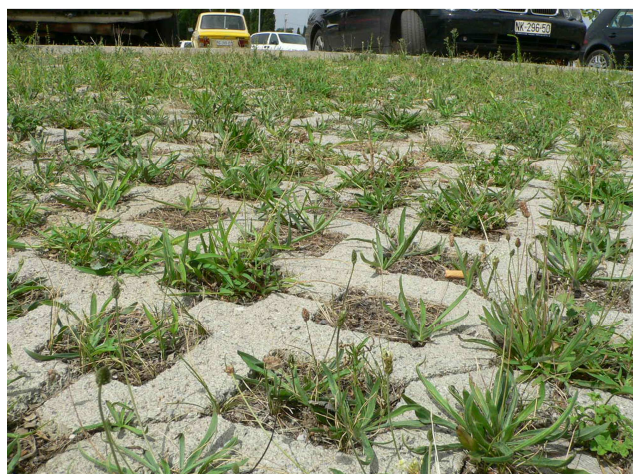
Figure 69. Parking lot (near Sports Centre).
