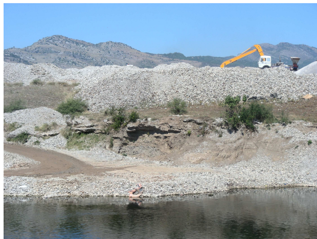
Figure 3. Exploitation of gravel (bank of Morača River-Kokotski ovčar).
