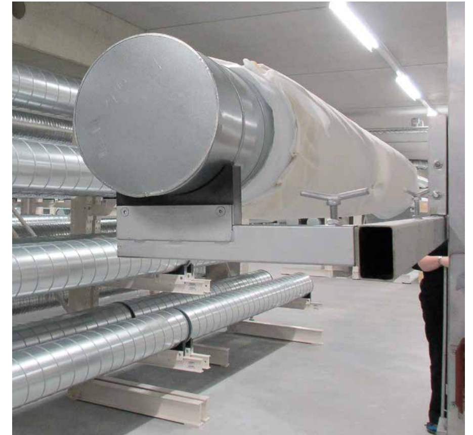
Fig. 15: Lifting apparatus in action.
