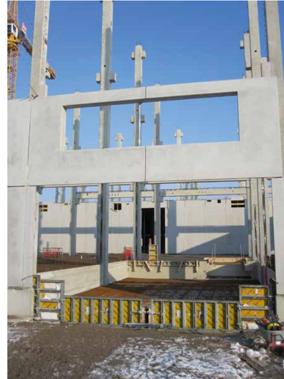
Fig. 3: Facade construction units with gaps for the windows.
