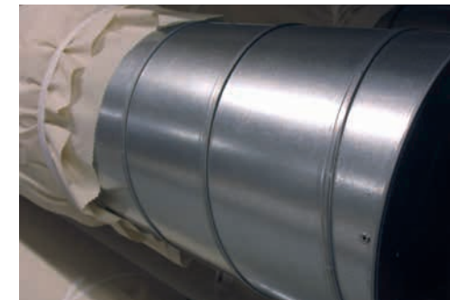
Fig. 5: Handling surface of the folded spiral-seam pipe.
