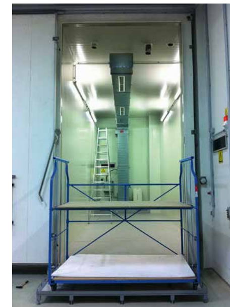
Fig. 70: View of the anoxic nitrogen treatment chamber of the Kunsthistorisches Museum Vienna.
