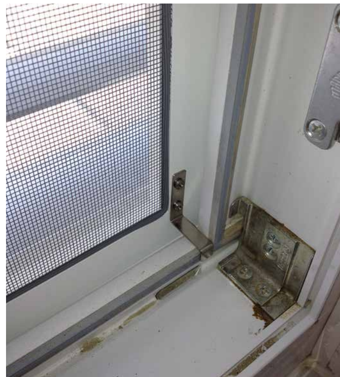
Fig. 15: Insect screens on the windows of the new storage facility.
