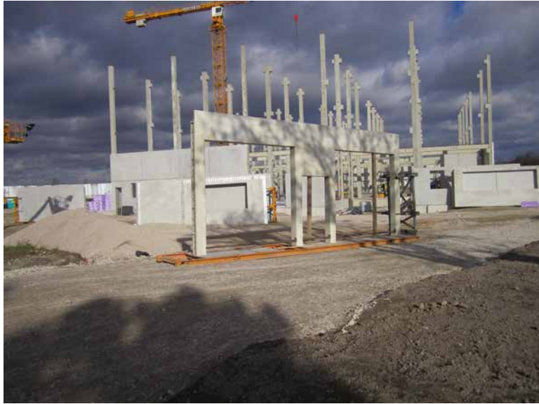
Fig. 2: Prefabricated industrial construction units contributed substantially to the short construction time.
