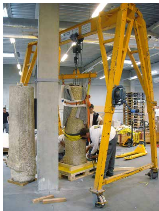
Fig. 76 a Transfer of milestones with a gantry crane and forklift.
