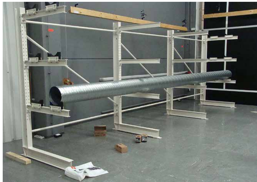
Fig. 63: Inzersdorf storage facility: Assembly of a prototype for the column-free rack from the company Magista Systems/Van Keulen Interieurbouw for storage of the Kunstammer tapestries.
