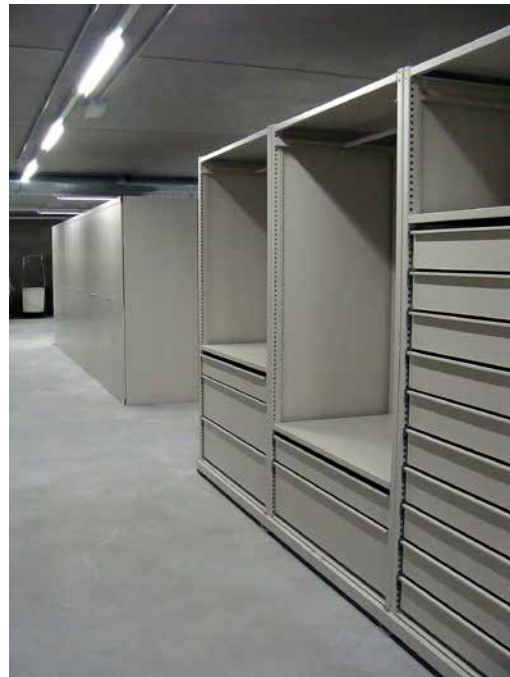
Fig. 56: Powder-coated steel cabinets from the company Magista Systems/Van Keulen Interieurbouw with variable interior fittings during assembly.
