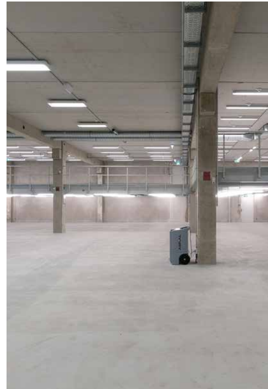
Fig. 7: The installation of intermediary steel platforms made it possible to optimise the use of the ceiling height.
