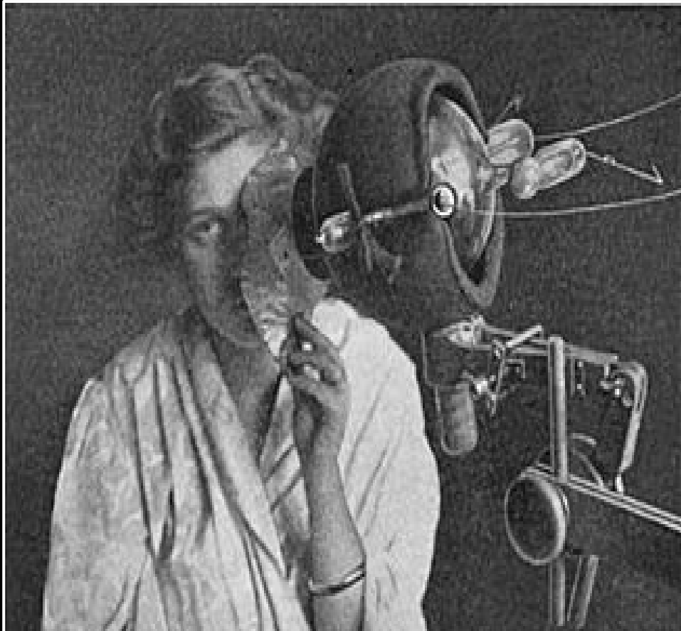
X-ray apparatus used for treatment of epithelioma of the face, 1915. The tube is in a localizing shield, and a perforated sheet of metal is securely fashioned to the surface by adhesive plaster
