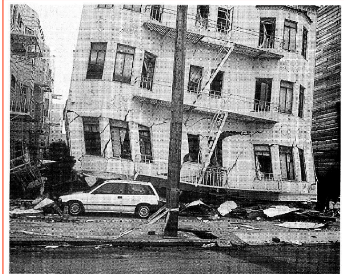
Figure 4.26 (a) Water-saturated sediment usually rests quietly. However, when seismic waves shake, sand grains and water can form a slurry and flow as a liquid. When earth materials liquefy, building foundations may split and buildings may fail. (b) A typical Marina District building collapse. Three residential stories sat above a soft first story used for car parking; now, the four-story building is three-stories tall. Photo courtesy of Dames and Moore.
