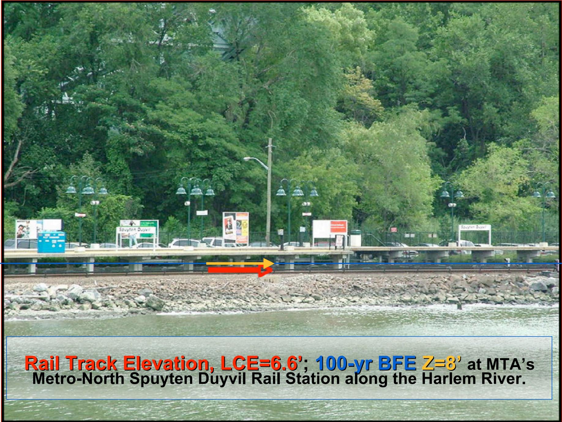
**Rail Track Elevation, LCE=6.6'; 100-yr BFE Z=8'** at MTA's Metro-North Spuyten Duyvil Rail Station along the Harlem River.
