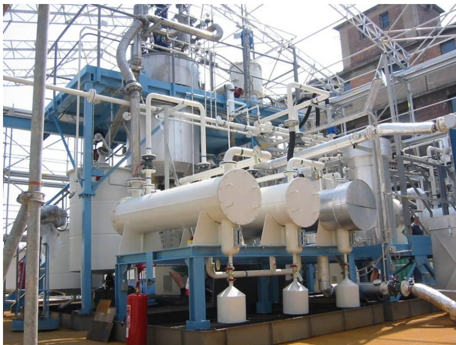
Pilot Plant Erection, Spolana
