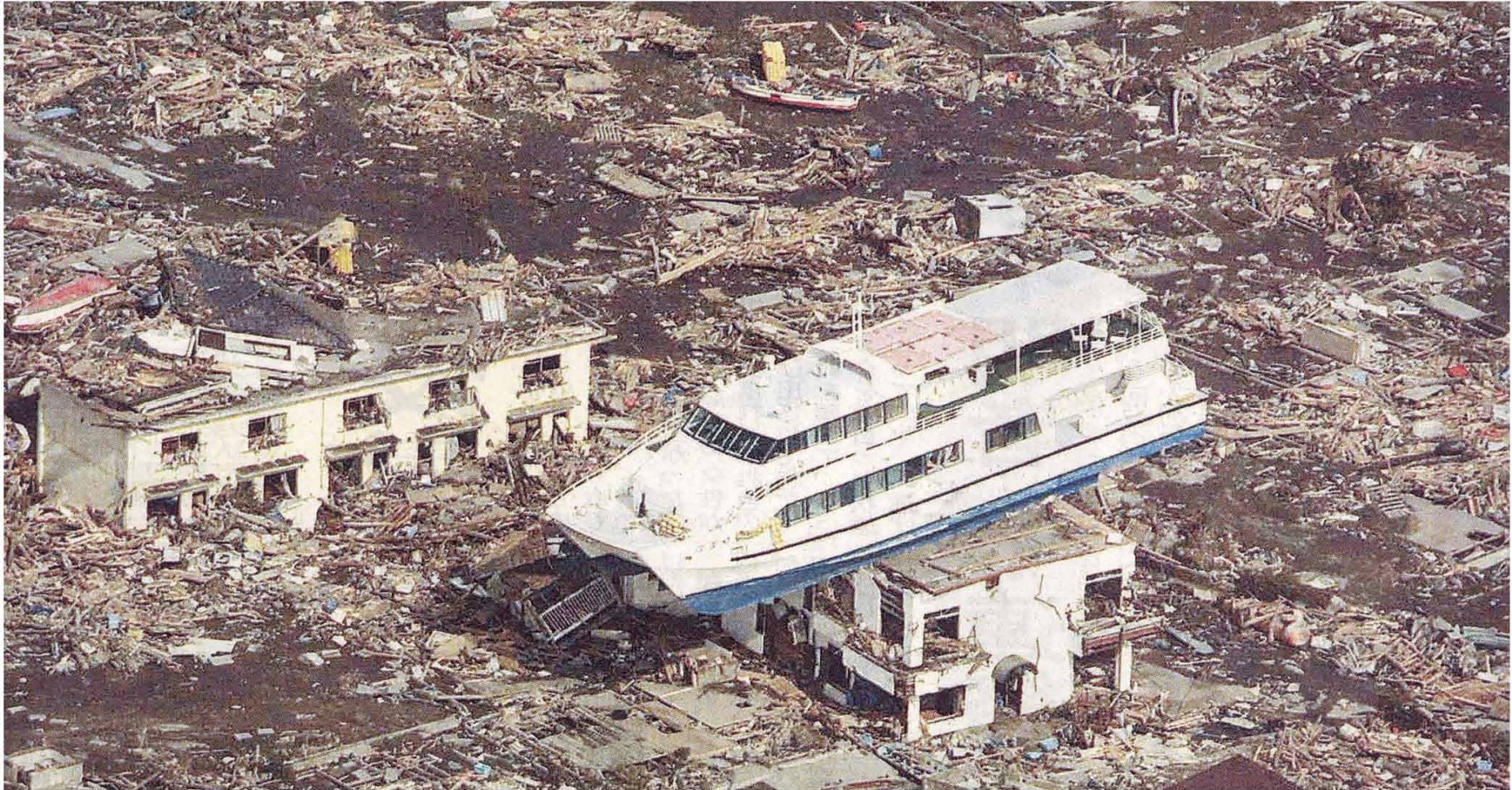
Fig.2b A big boat flown on the roof of a building in Otuchi Town, Iwate Prefecture
