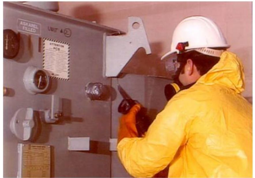
Had to be cut apart by hand
