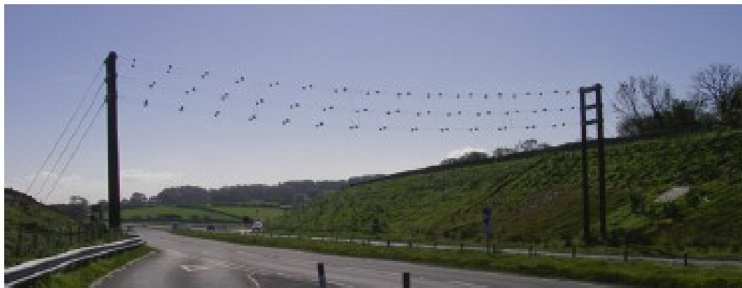
Fig. 3.5 The most common bat gantry design in the UK—steel wires with plastic spheres at intervals that are intended to be acoustic guides for bats
