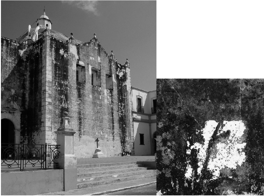
FIGURE 5.4 A thin black crust on Campeche cathedral, Mexico. Smaller photo shows close-up. Dark brown branching filamentous cyanobacteria were the main component (authors' unpublished observations).
