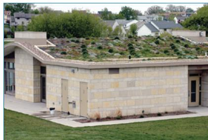
Both cool and green roofs lower surface and air temperatures and reduce summertime peak and overall energy demand. The extent of the energy savings varies depending on factors including the local climate, attic ventilation and insulation levels, and—particularly for green roofs—the design and maintenance of the roof.
