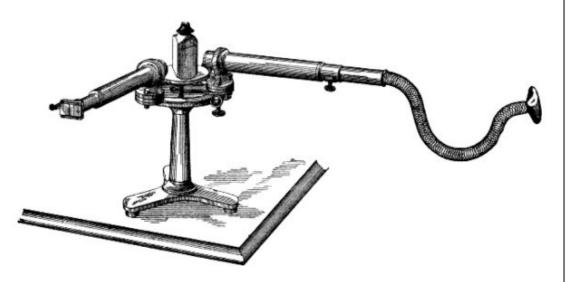
In 1881 A.G. Bell proposed a *spectrophone* "for the purpose of examination of the absorption spectra of bodies in those portio of the spectrum that are invisible".
