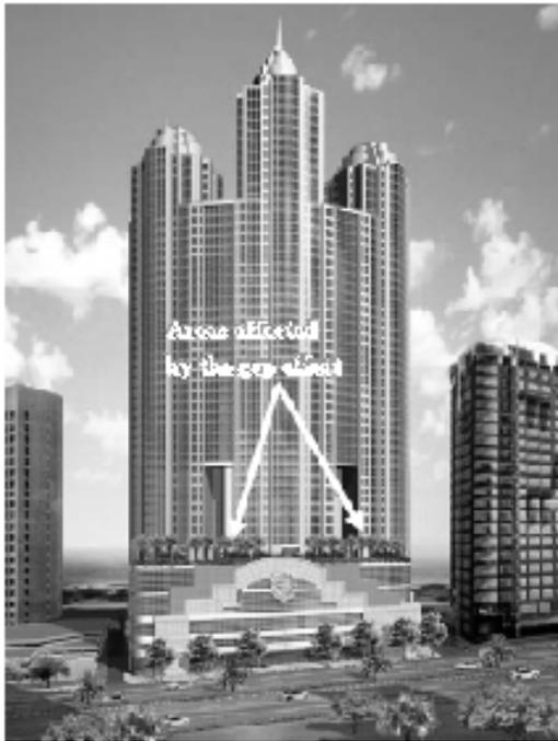
**Fig. 7: The Abu Dhabi development with the areas affected by the gap effect indicated**
