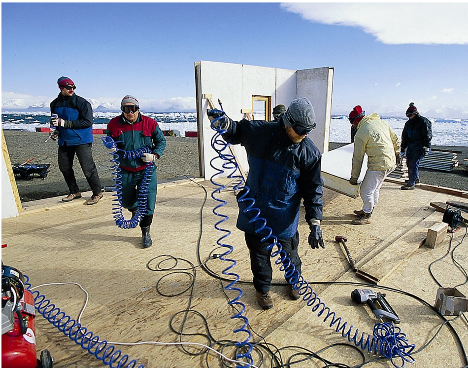
Fig. 4. K-Kontrol construction system is based on sandwich panels made of two OSB chipboards and inner insulation layer. © Photo: H. Adámek.
