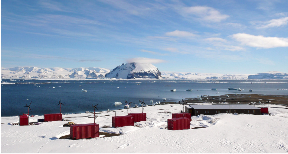
Fig. 9. Significant part of technical systems and storages are placed in standard 20-feet containers. © Photo: K. Láška.
