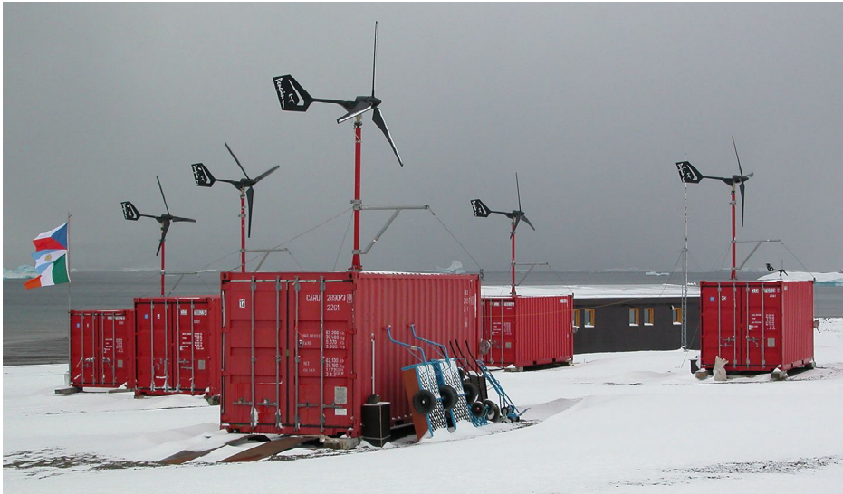
Fig. 13. A group of wind turbines (AP1500) facing SE wind. © Photo: K. Láska.
