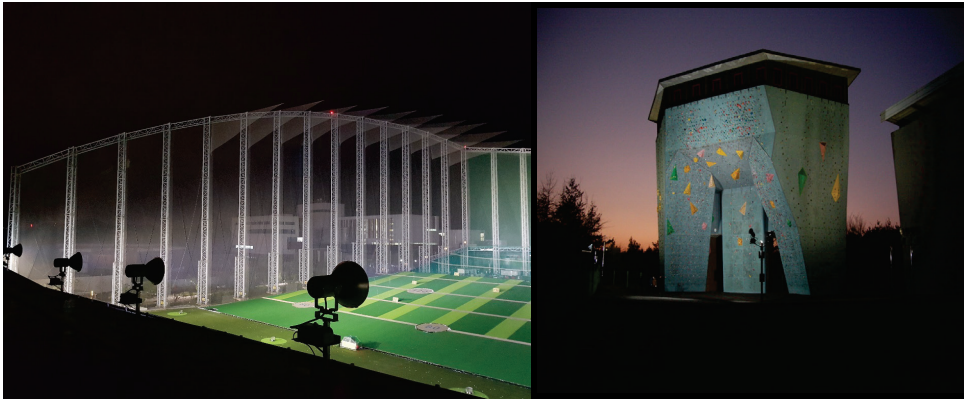
Figure 9. Plasma lights are used for sports lighting. A golf driving range is well illuminated by plasma lights. The flying ball can be clearly visible at a distance of over 200 m away (L). A rock climbing wall is illuminated at night (R).
