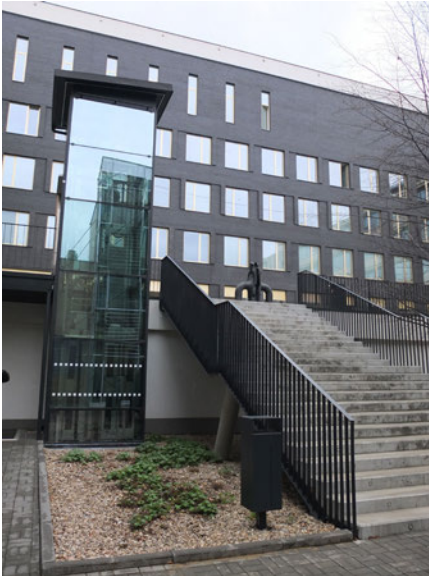
Figure 4.2 Exterior lift helping to overcome height differences at Masaryk University in Brno (photo: Z. Čerešňová)
