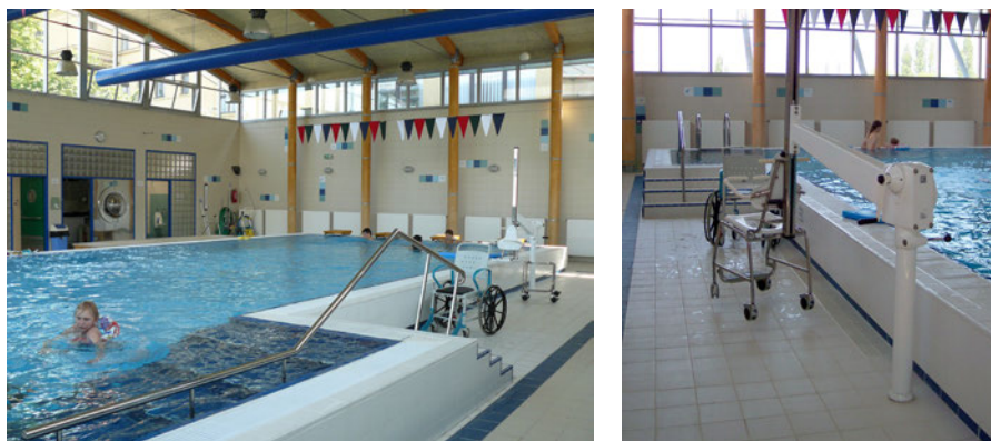
Figure 4.15 Swimming pool with multiple options to access the pool (transfer steps, fixed and mobile lifting devices), Jedlička's institute in Prague (photo: L. Rollová)
