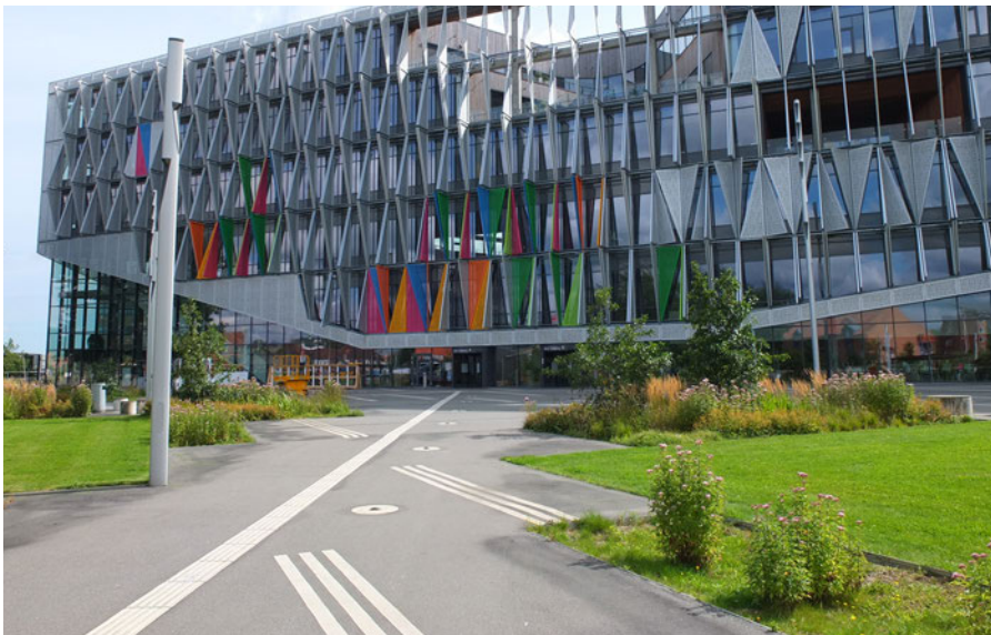
Figure 4.4 Artificial guiding line (embossed tiles) leading to the main entrance to Kolding Campus, University of Southern Denmark, Henning Larsen Architects (photo: Z. Čerešňová)
