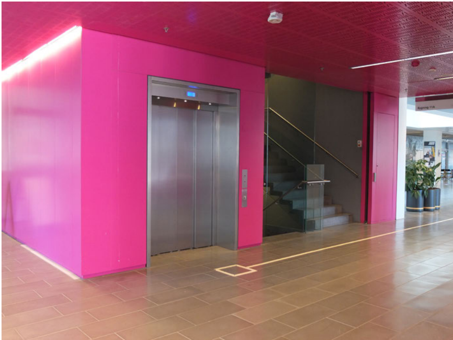
Figure 5.27 Tactile guiding lines and colour contrasts in circulation spaces, University of Copenhagen, Arkitema Architects (Photo by Z. Čerešňová)
