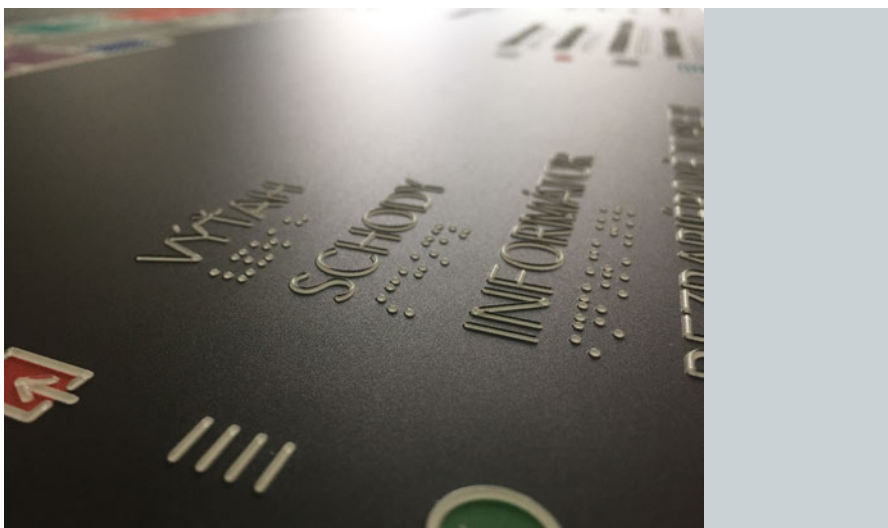
Figure 5.29 Braille and Raised Characters on the tactile floor plan of the Faculty of Architecture, Slovak University of Technology in Bratislava (Photo by A. Kubica)
