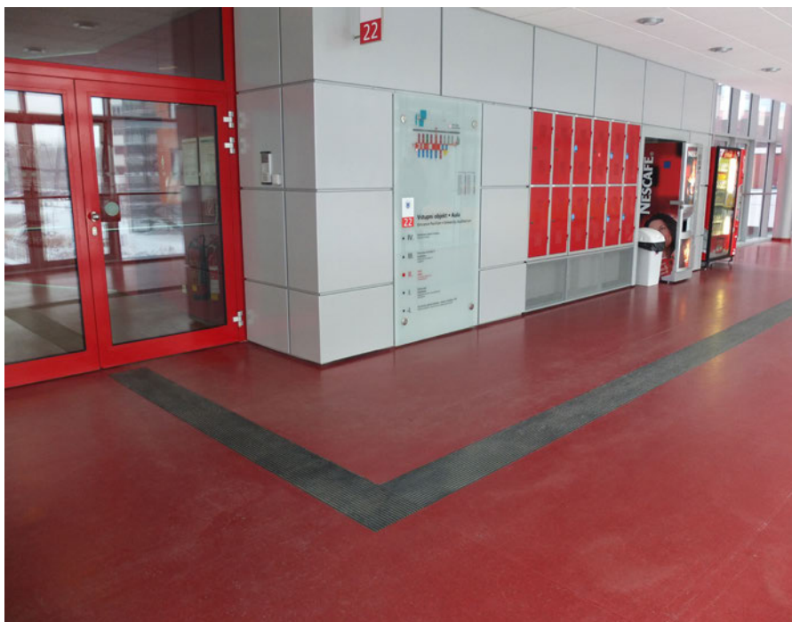
Figure 5.26 Tactile guiding lines and colour contrasts in circulation spaces, Masaryk University in Brno, architects: A PLUS (Photo by Z. Čerešňová)
