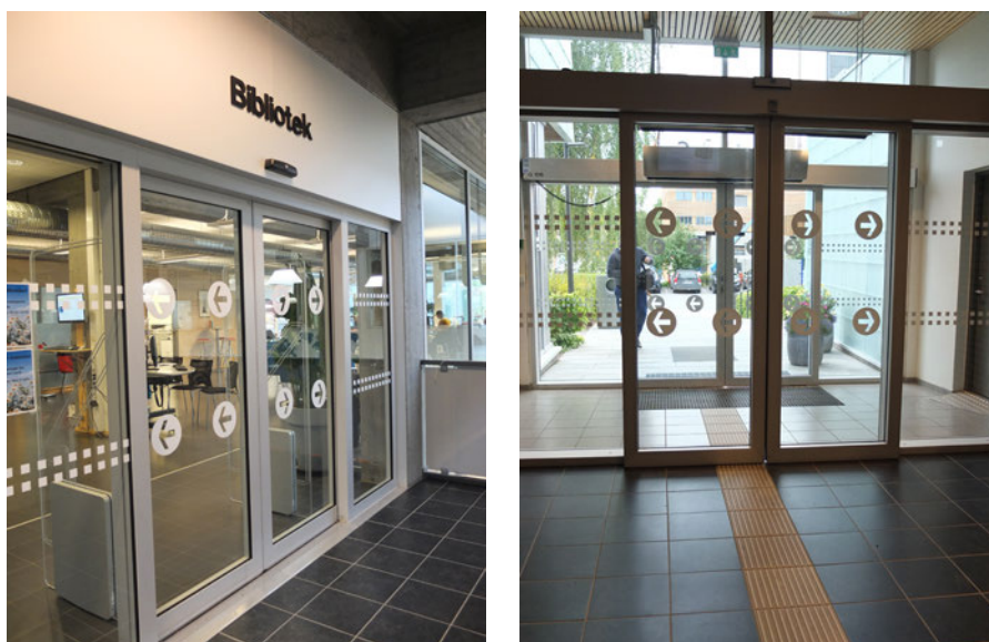
Figure 5.1 a, b Colour contrasting signs on the entrance doors and tactile guiding lines in the entrance area (Photo by Z. Čerešňová)
