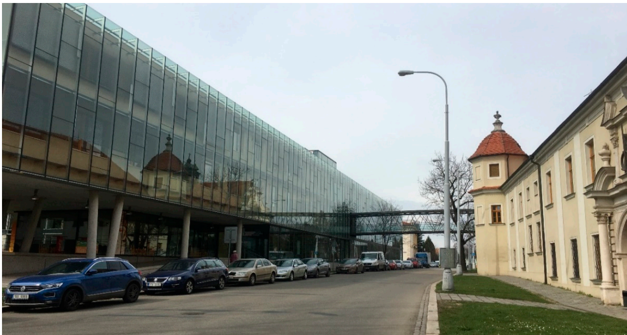
Figure 8. Bridge connection of the western part of the site with the eastern historical part with contrasting architectural styles (Photo: K. Charvátová).
