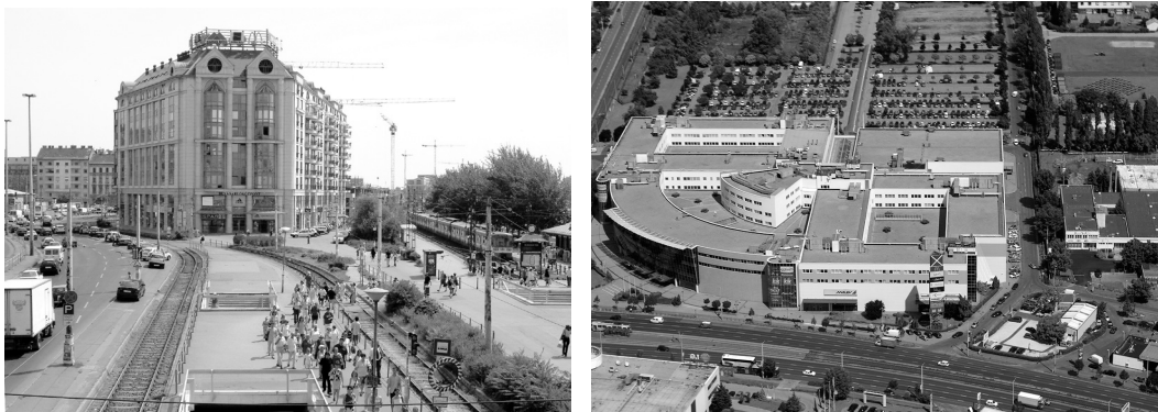
Fig. 4.15: Duna Ház and the Lurdy Ház the losers of the market of shopping centres
