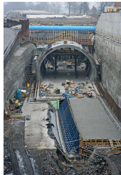
Tunnel construction in Troy, Prague.
