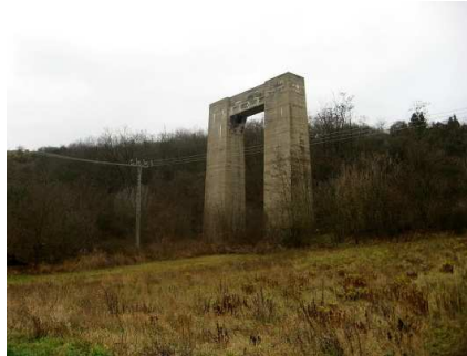
Motorway pillar near the Brno Dam
