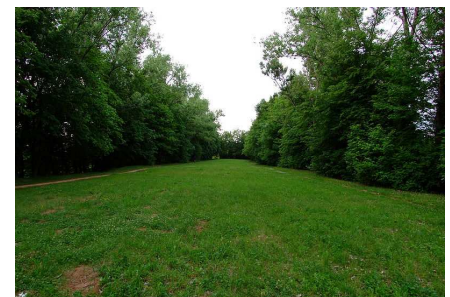
Unfinished part of the motorway bank in Brno-Bystrc
