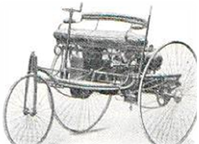
Benz's three-wheeled carriage powered by petrol.
